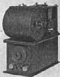
Fig. 9. Tesla Transformer, with mercury interrupter
