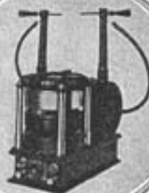
Fig. 8. Tesla Transformer with rotary break for wireless
